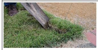
4. Determine how far to raise the head and carefully cut the riser extension.
