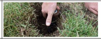
9. Attach a flush nozzle and briefly turn the system on to clean out the sprinkler body.
