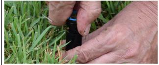
Remove the nozzle and the filter.
