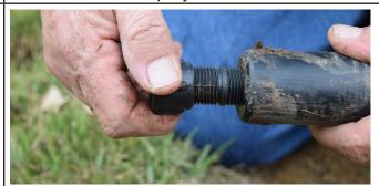
8. Screw the female end onto the funny pipe elbow or existing nipple.
