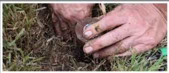
For sprays that are throwing the wrong direction, simply take hold of the spray stem and gently "ratchet it around" to the correct position. The ratchet sound you hear won't damage the spray head.
