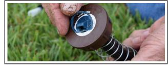
If your spray heads are old, you might dig up the old spray head and replace it with a pressure-regulated head. Pressure-regulated spray bodies are available in three, four, six and 12-inch models.
