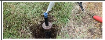
10. Replace the soil and nozzle. Make sure the spray body is straight and check your work.
