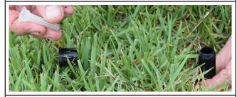
Hold the stem with one hand, drop in the new filter and screw on the new rotating spray nozzle. Turn on the irrigation system and check your work.
