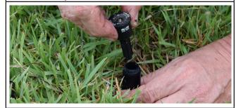
Over time, sprinkler heads get out of adjustment from tree roots, mowing equipment, settling of soil, kids and many other factors. When you replace clogged or broken nozzles, make certain you replace the nozzle with the exact same brand and size or replace the entire zone with waterconserving nozzles.
