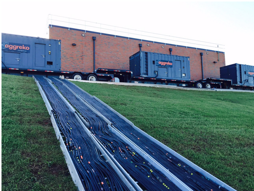
Three temporary diesel generators provide power to the Draper water treatment plant via 600 feet of cable.
