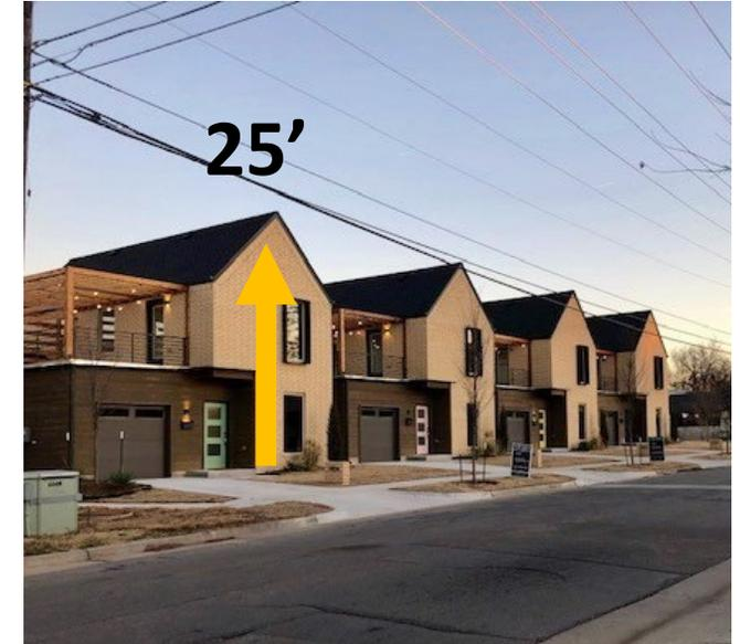
**Building Height: The vertical distance from grade to the highest point of a coping of a flat roof, or to the deck line of a mansard roof, or to the average height of the highest gable of a pitched or hip roof**
